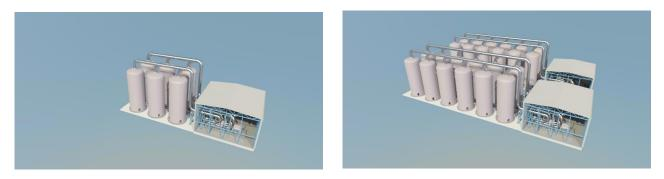
The GridScale energy storage consists of one or more sets of steel tanks filled with crushed stone. Charging and discharging is obtained using a system of compressors and turbines. Both the number of sets of storage tanks and the number of turbine units may vary depending on the length of the discharge cycle wanted as well as the electrical power wanted.
