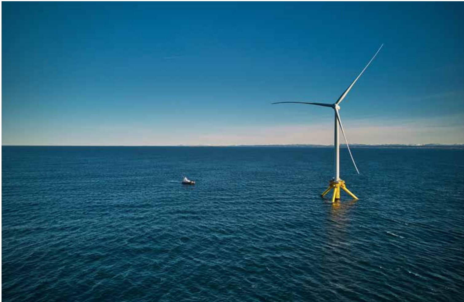
The TetraSpar Demonstrator in operation: The world's first fully industrialized offshore foundation operating at 200m water depth at the METCentre test site off the coast of Karmøy, Norway.
