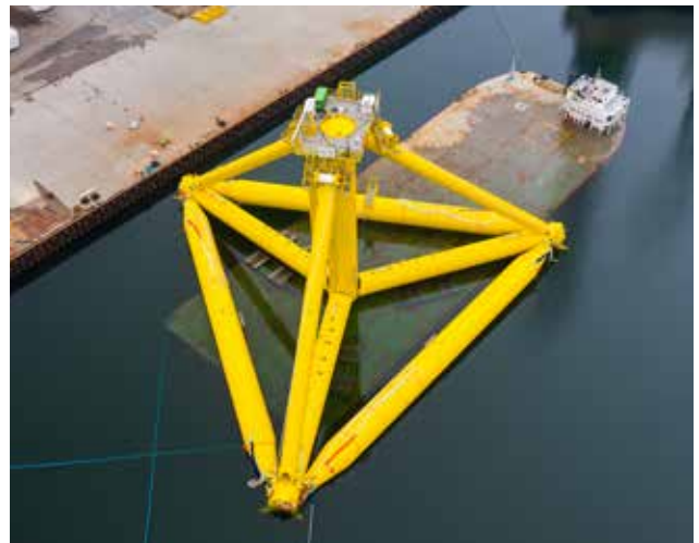
Launch of the TetraSpar Demonstrator using semisubmersible BOA Barge.
